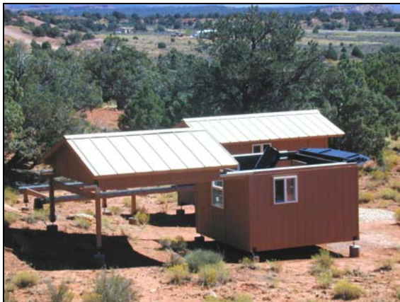
Figure 2. Completed Vermillion Cliffs Observatory – Venus Building with Vermillion Cliffs Observatory in the background.
