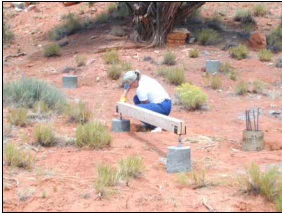
Figure 1. Placing the first floor support beam.
