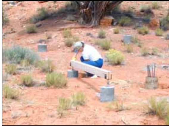
Figure 1. Placing the first floor support beam.
